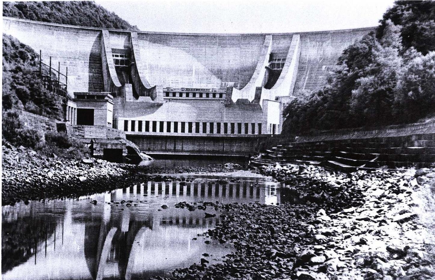
**EQUIPEMENT HYDRAULIQUE :** IL Y A VINGT ANS, EN 1951, ÉTAIT MIS EN SERVICE AU CHASTANG LE PREMIER GRAND OUVRAGE ENTIÈREMENT RÉALISÉ PAR EDF SUR LA DORDOGNE. LE BARRAGE, HAUT DE 80 MÈTRES, CRÉE UNE RETENUE DE 180 MILLIONS DE M<sup>3</sup> D'EAU QUI ALIMENTE UNE USINE D'UNE PUISSANCE DE 270 MW.
