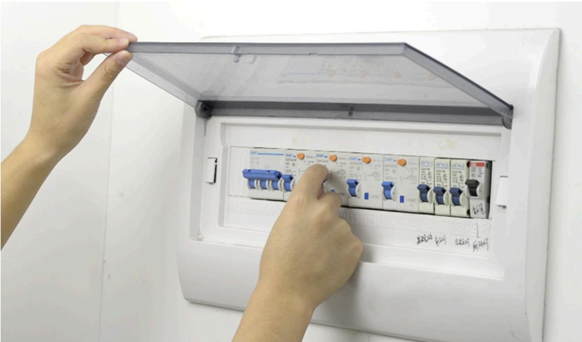
Confirm that the power is off by using the voltage tester to check the Live wire and terminal. No electricity should be present.
