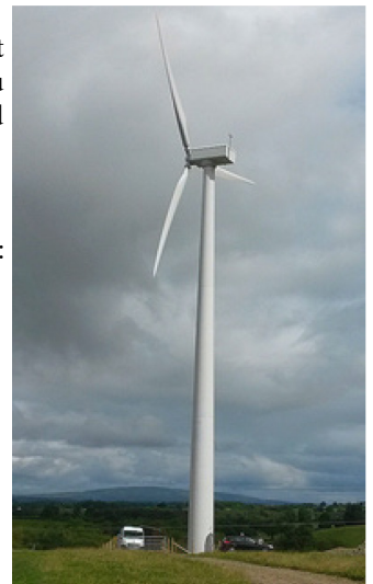
Figure 14 : Eolienne WTN 250 kW
