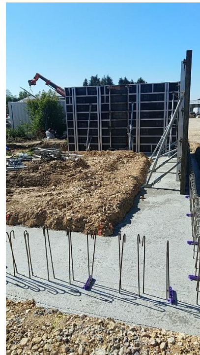
Pose des coffrages NOE top
