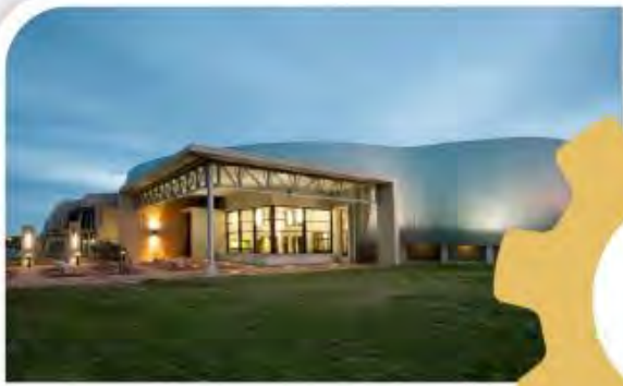
New Engineering Building
