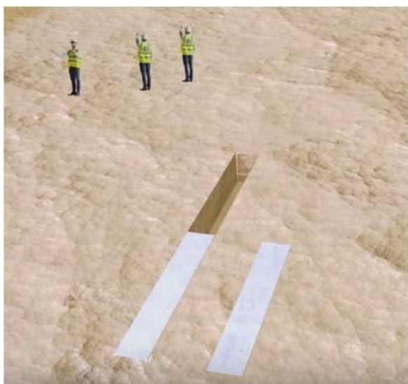
Figure 2 : Construction des murettes guides, source [2]
